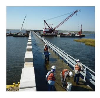
The significantly lower modulus and increased tensile elongation of T-70 provides better compatibility with moving cracks and thermal stresses.
